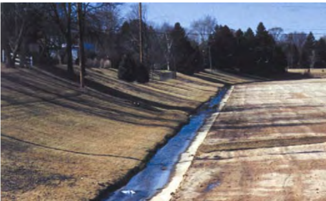
Churchill Lane Detention Basin
